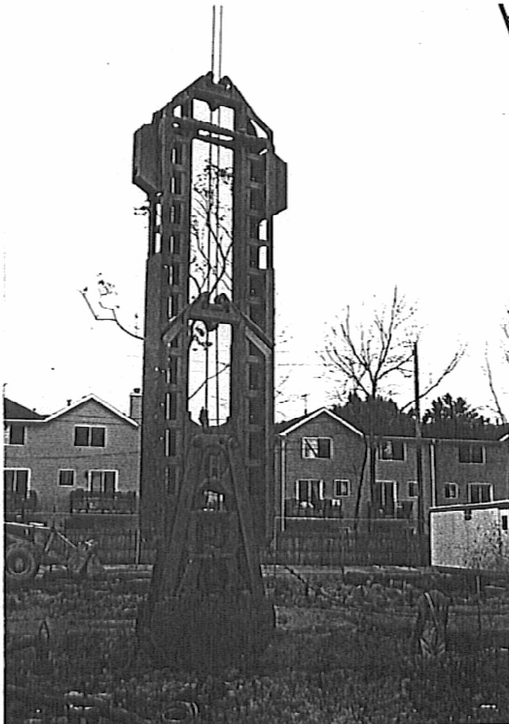
Photograph 2. Cable suspended excavating grab, showing long frame extension.
