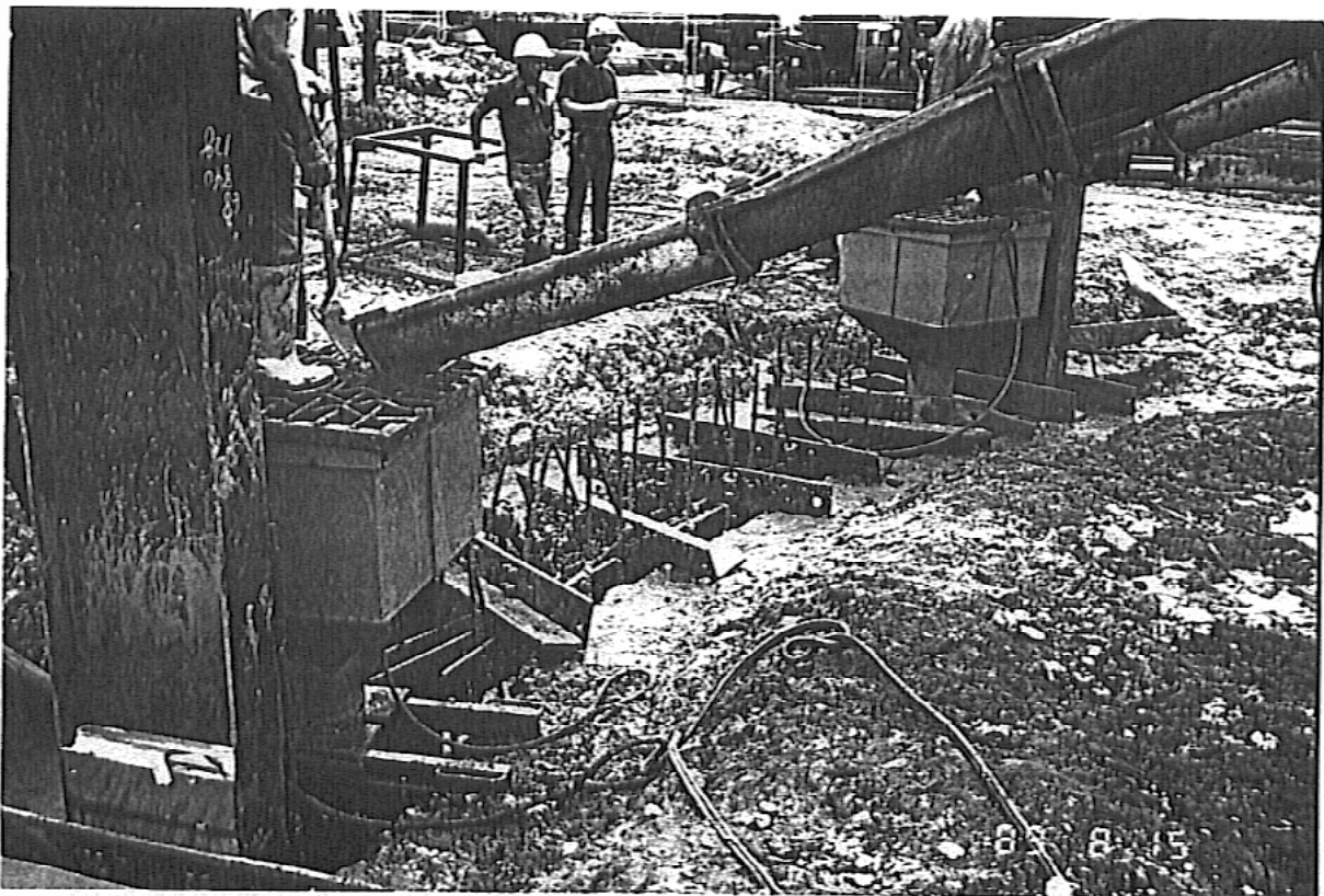
Photograph 4. (Below) Tremie concreting a Primary panel using two lines.
