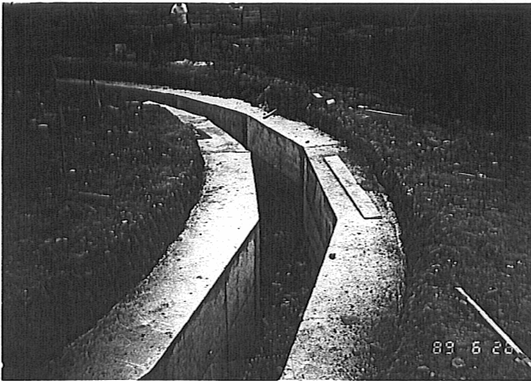
Photograph 1. Guide walls, prior to slurry wall excavation
